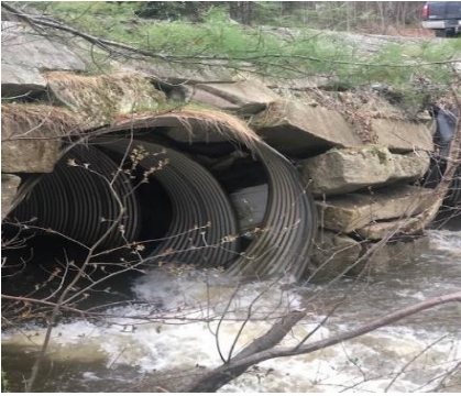
East Sandy River Road Culvert
