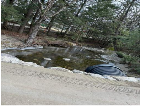
Pattie Brook Culvert Fixed
