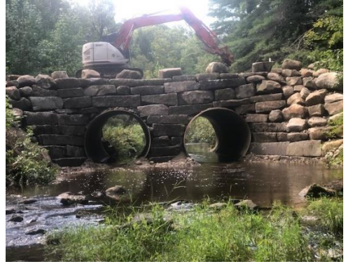
East Sandy River Road Culver Repair
