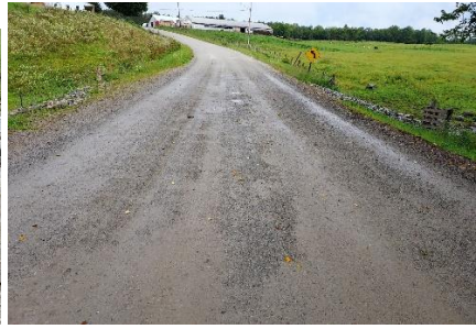
Elm Street Culvert Repaired
