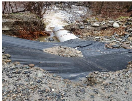
Rome Road Culvert
