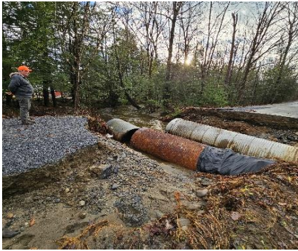
Pattee Brook Culvert
