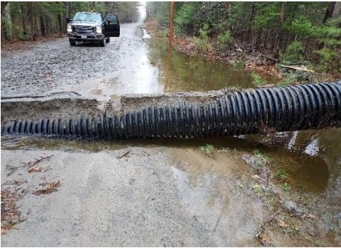
Corson Road Culvert
