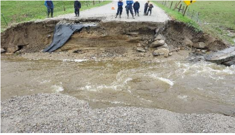
Elm Street Culvert
