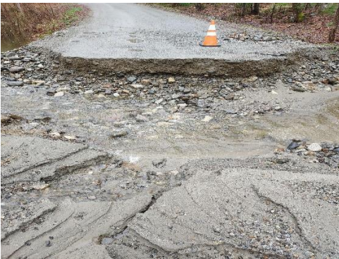
Decker Road Culvert
