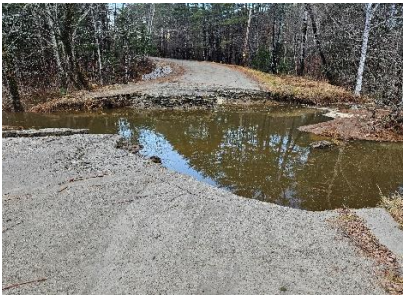
Indian Stream Culvert
