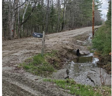
Corson Road Culvert Repaired
