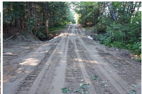
West Sandy River Road Culvert Fixed
