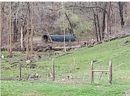
Elm Street Culvert Downstream
