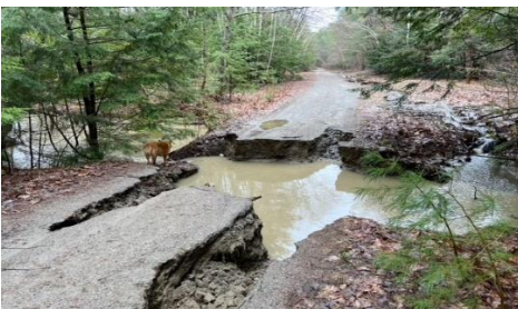
West Sandy River Road Culvert
