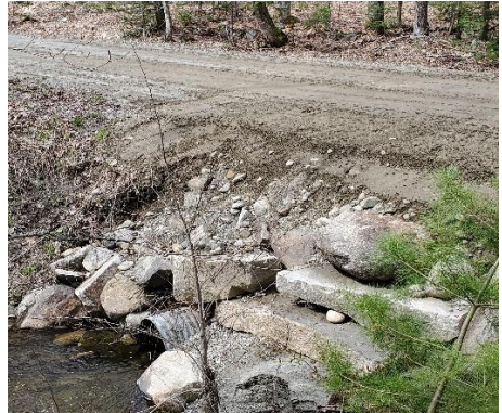
Decker Road Culvert Fixed
